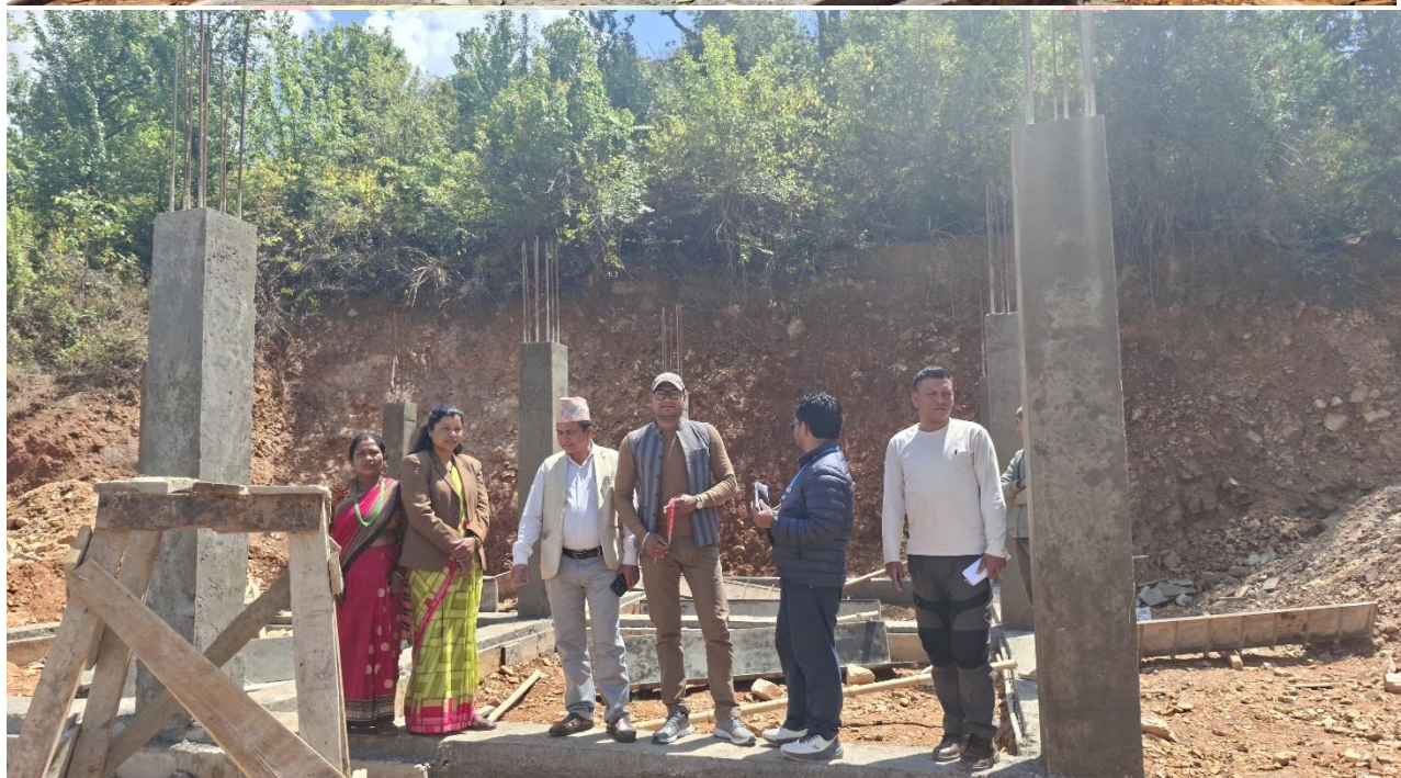
CONSTRUCTION OF WARD OFFICE WARD NO.10 MANGALSEN-10, ACHHAM
