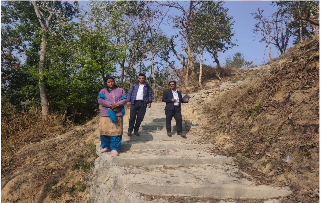
TOLAGADA KAILASHKHOLA MALAMI PADMARG NIRMAN MANGALSEN-04,ACHHAM
